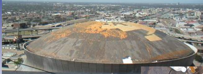
• Failure of roofing membrane on Superdome
