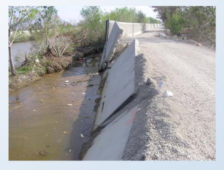
• Failure was likely triggered by erosion and piping of soil due to underseepage according to IPET study.
