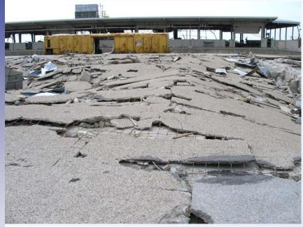
• Collapse of wharf at Port of Gulfport due to pile failure.
