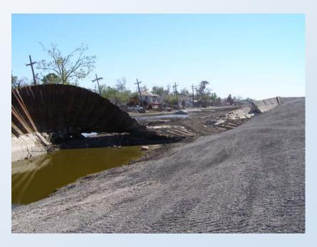
Rotational failure of floodwall-sheetpile due to overtopping and scour on protected side of levee.
